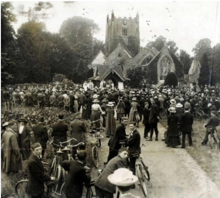
After the fire at Wargrave church: an open-air service
