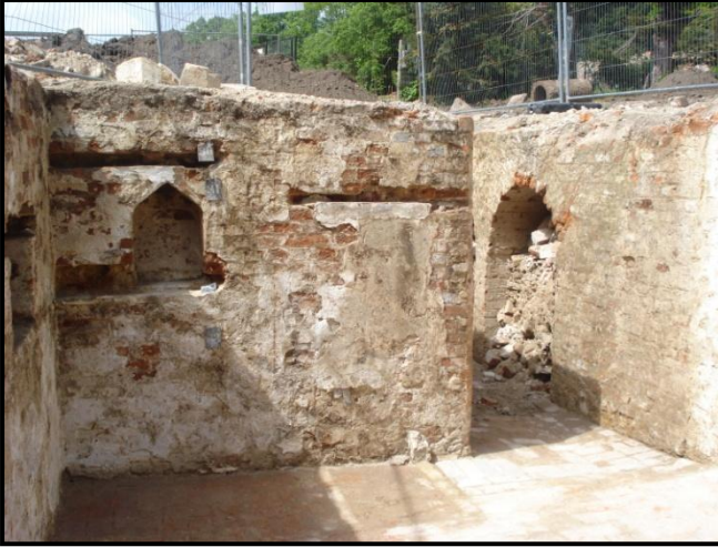
The Old Rectory cellars uncovered unexpectedly during the 2009 restoration! The Regency wine cellar is in the foreground and the vaulted Tudor beer cellars are in the background (right). These have now been covered up again, and are located under the house footprint.
